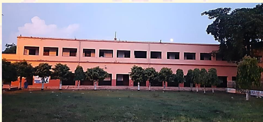
Rampurhat College: Classrooms
